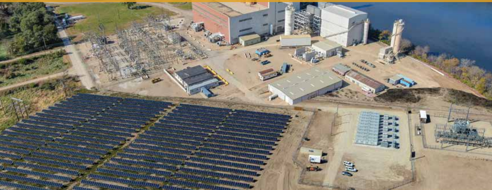
Above: This concept rendering shows how the legacy Hennepin power station which closed in 2019, would be repurposed to have utility-scale solar (20 MW+) and energy storage built at the site. Detailed plans have been completed and shared with the grid operator.
